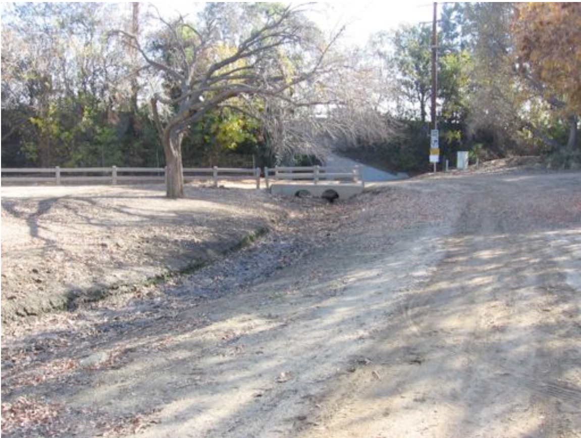
Fig. 3. Dirt culvert in Crystal Springs area (drains to Los Angeles River) which could be restored to a more natural state. Photographed Dec. 2007 by Daniel S. Cooper.
