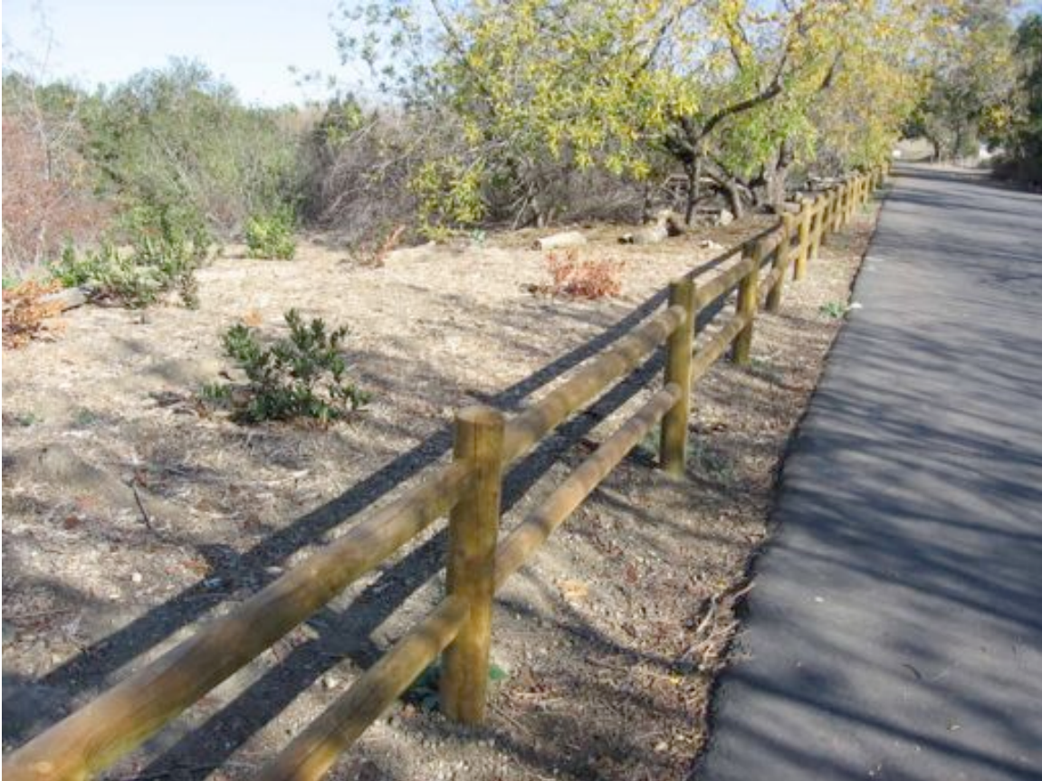
Fig. 2. Example of solid, naturalistic (wooden) fencing between a habitat restoration area and road at Debs Park (in Highland Park, Los Angeles). Photographed Jan. 2008 by Daniel S. Cooper.
